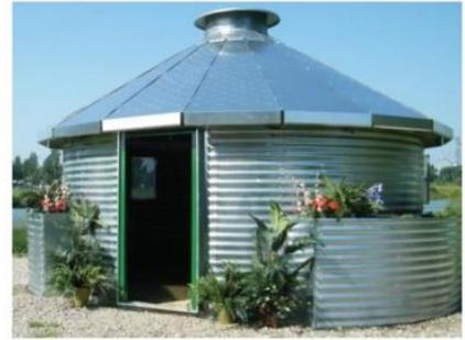
The Safe T Home can withstand the devastating hurricanes and earthquakes that have plagued Haiti over the last decade. In fact, in 2016 when Hurricane Matthew hit Haiti with 145 mph winds, all 200 of the grain bin homes that were built there remained strong with only minimal damage, while only 10% of the traditional homes remained.
