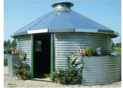
The Safe T Home can withstand the devastating hurricanes and earthquakes that have plagued Haiti over the last decade. In fact, in 2016 when Hurricane Matthew hit Haiti with 145 mph winds, all 200 of the grain bin homes that were built there remained strong with only minimal damage, while only 10% of the traditional homes remained.
